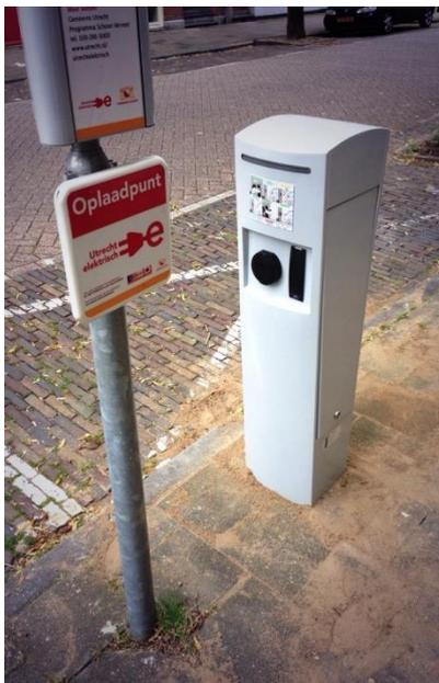
*Figure 6: AC V2G station from General Electric*
